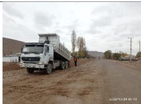
Photos 27. Subgrade material fill (2nd layer) km 69+820-70+400 LHS
