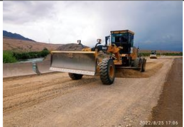
Photos 16. Subbase construction km 11+320-11+380
