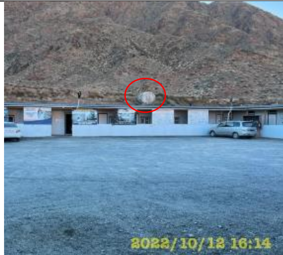
Photos 45. Domestic water tank (built-in).
