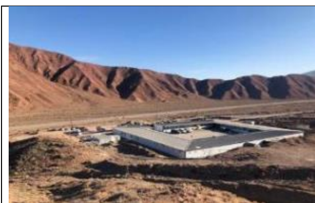
Photos 36. General view of the camp Lot 1 km 16 + 100 (RS).
