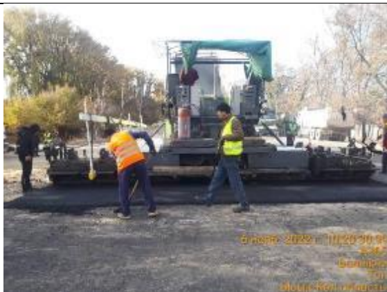
Photos 19 binder km 2+100-2+600 LHS
