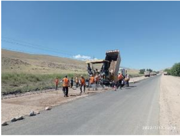
Photos 28. Paving of base material km 85+248 RHS
