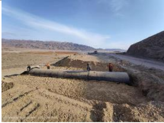
Photos 13. Backfill pipe 3rd layer km. 40+811
