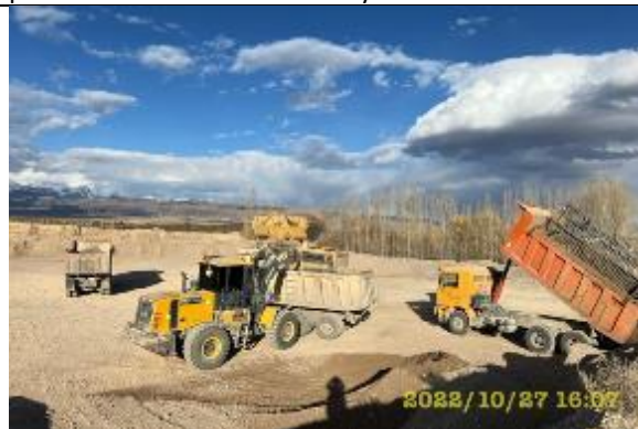
Photos 72. Pit development at km 75+400
