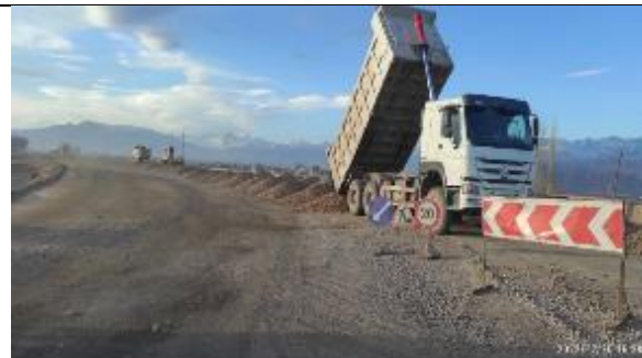
Photos 25. Backfilling of 3 layers of embankment 65+520-65+620
