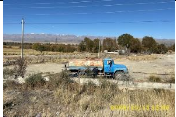
Photos 77. Lot 2. Water intake
