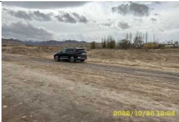
Photos 78. Behind the bypass road reclaimed unusable soil dump located at km.65+520
