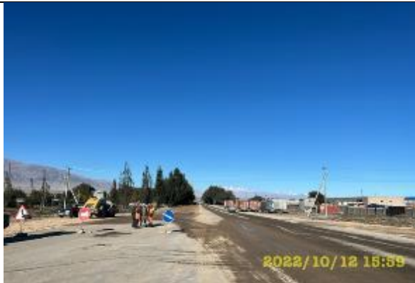
Photos 60 Lot 1. Watering of unpaved sections of the road km. 03+200.
