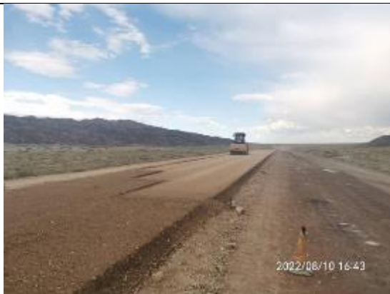
Photos 17. Base layer km 33+000 - km 33+340 RHS.
