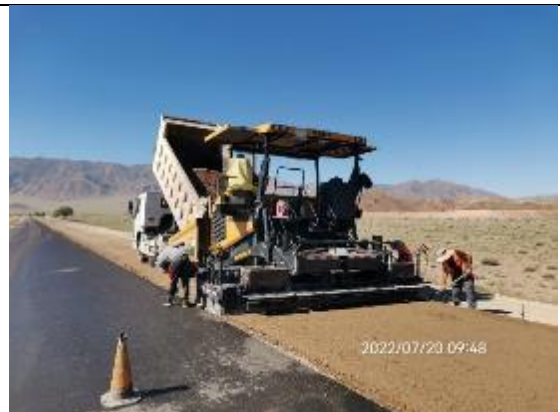
Photos 18. Paving base in the 21+500-22+000 RHS section.
