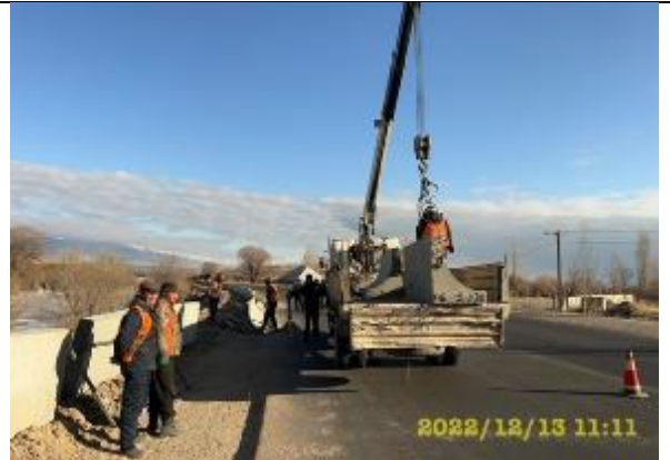
Photos 67. Installation of parapets on Lot 1
