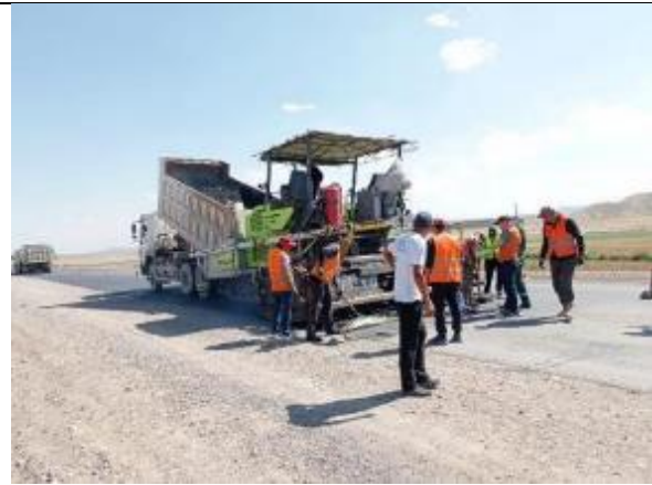
Photos 33. Construction of the SMA at km 79+600-80+100 RHS.
