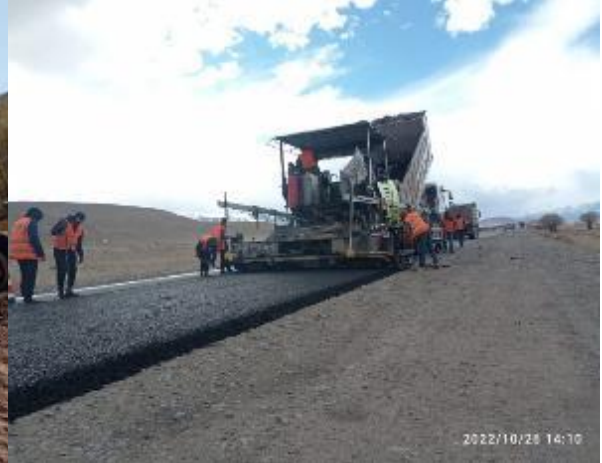
Photos 31. Construction of the SMA at km 81+675-82+000 RHS.
