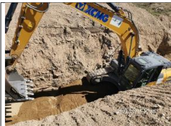
Photos 11. Pipe excavation at km 22+575
