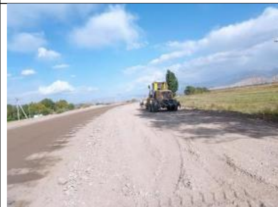
Photos 26. Planning sub-base material km 69+000-69+400 LHS
