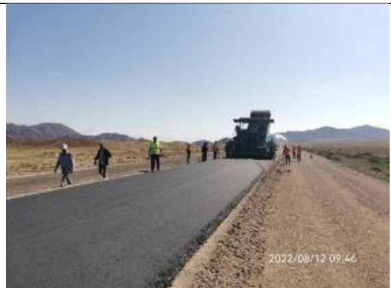
Photos 20. Paving binder at km 17+230 - km 17+500.
