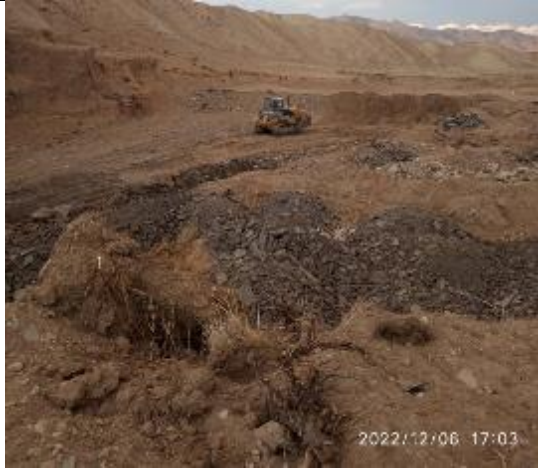
Photos 74. Planning of the old asphalt dump at km 89+500
