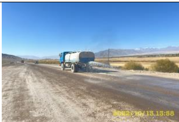
Photos 69. Watering along Lot-2 for dust control.
