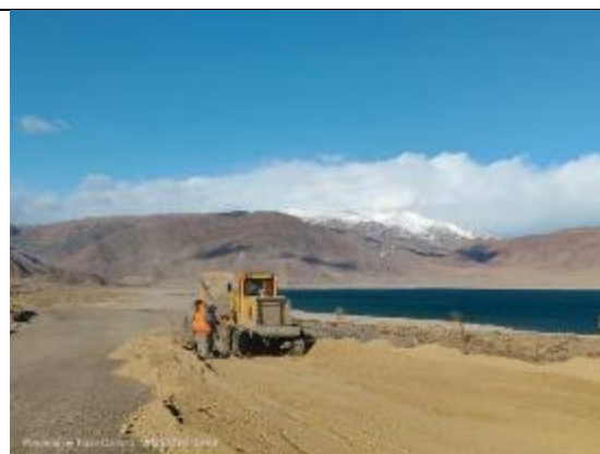
Photos 12. Backfill and leveling of embankment at km 36+000-36+500 RHS
