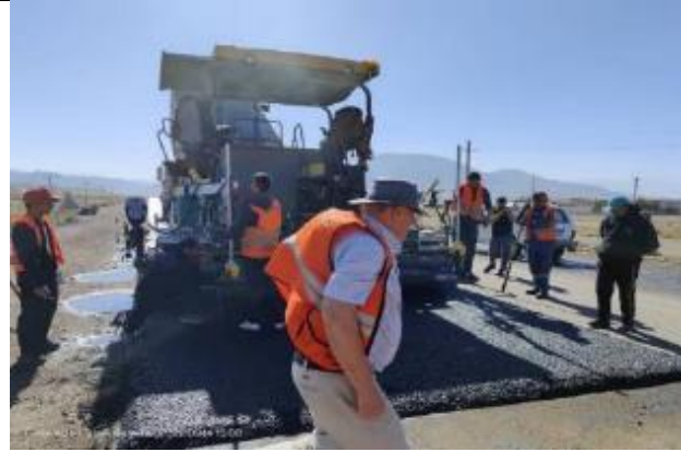
Photos 21. Paving SMA 3+140 LHS
