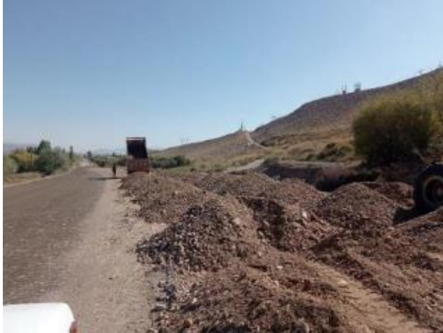
Photos 30. Backfill subgrade material at km 71+160-71+500 LHS.
