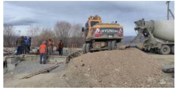
Photos 35. Concrete pouring of transition slab 1 km 68+044
