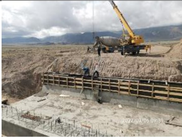
Photos 15. Concrete pouring of pipe wall km.22+255
