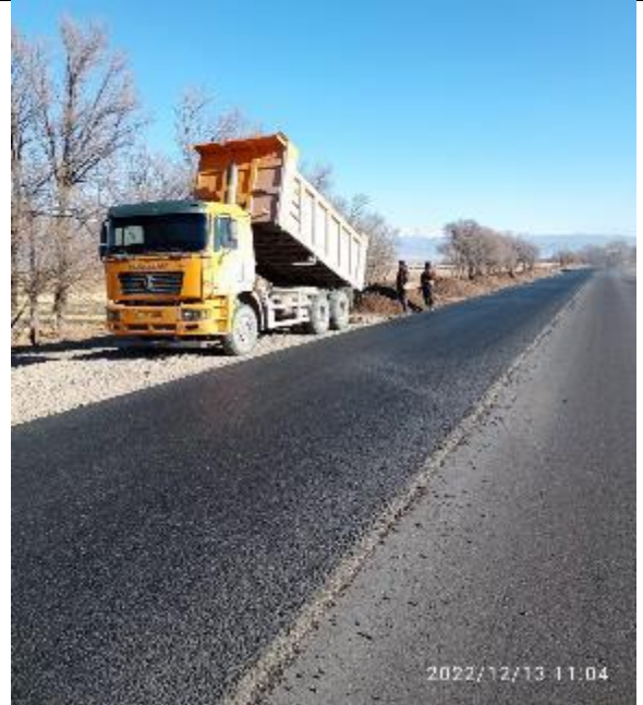
Photos 29. Installation of the top layer of roadsides of km 84+000-84+300 RHS.
