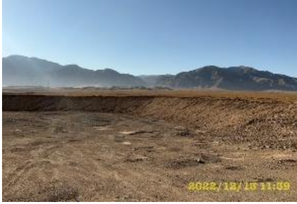
Photos 64. Performed technical reclamation of the quarry located at km.26+800 LHS.
