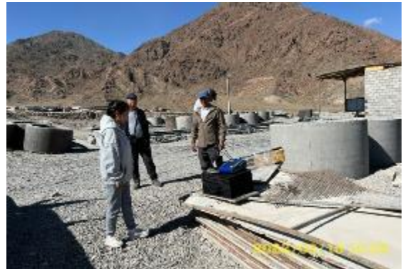
Photos 86. Lot 1. Production base. Noise and vibration measurements
