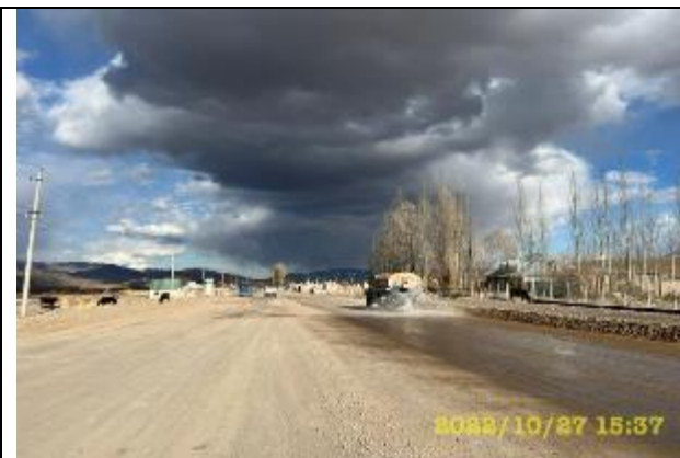
Photos 68. Watering unpaved areas of roads to prevent dust.
