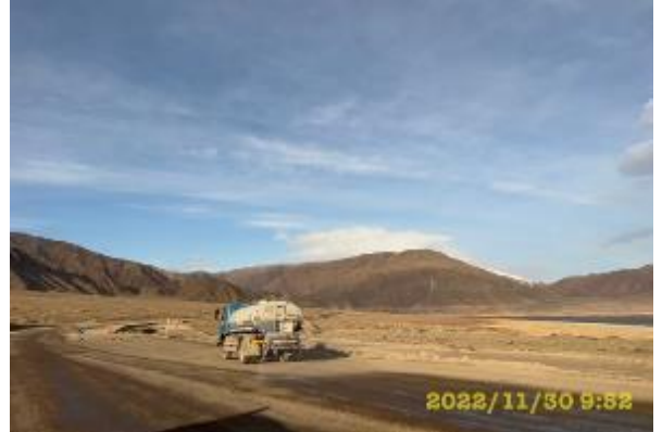
Photos 65. Lot 1. Irrigation of unpaved sections of the road km. 32+350
