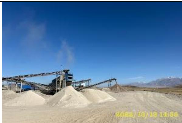
Photos 73. Stone Crusher in operation
