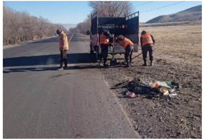
Photos 75. Sanitary cleaning of the project road
