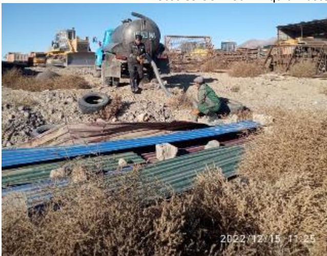
Photo 92. Lot 2. Liquid waste removal
