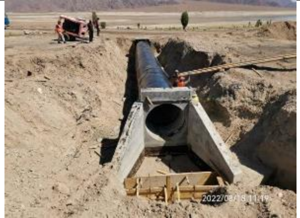
Photos 14. Completed culvert installation and waterproofing km 37+161
