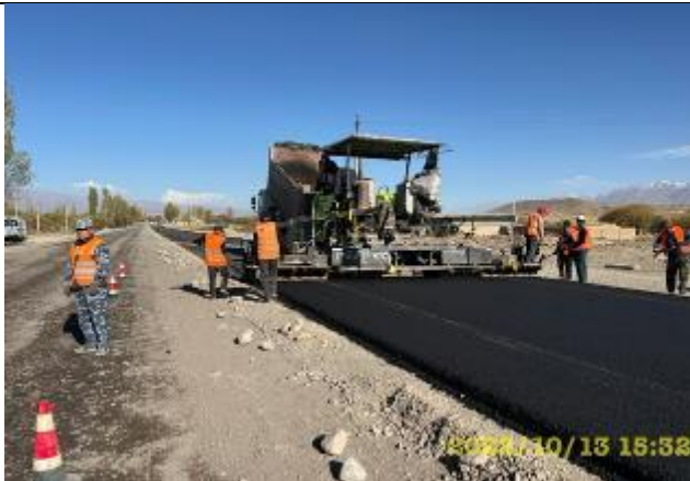
Photos 32. Laying of binder layer km 87+100
