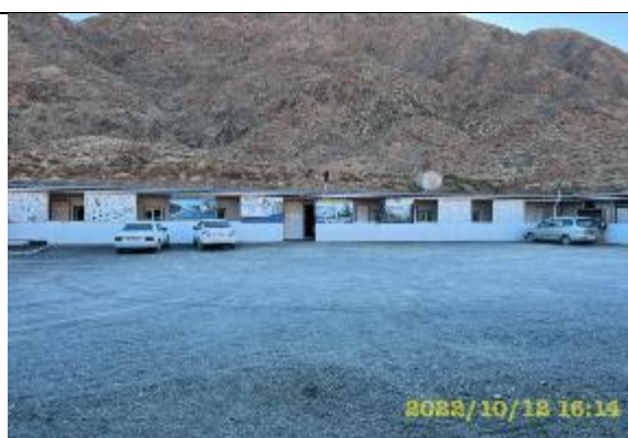
Photos 37. Lot 1 camp and parking lot at km 16 + 100 (RS)
