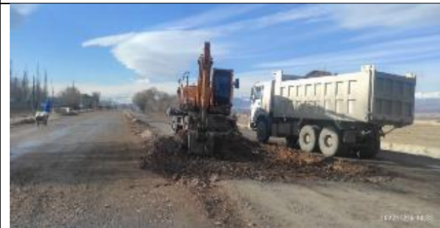
Photos 24. Grubbing the existing road surface at km 65+980 - km 66+220.
